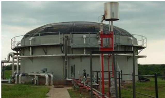
Anaerobic Sequencing Batch Reactor (ASBR) Digester Located on the Oklahoma State University
