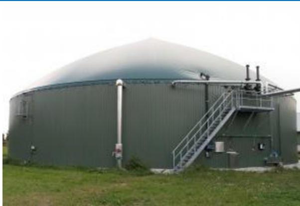
CSTR Plant in Langendorf (Germany) Fuente: www.ows.be
